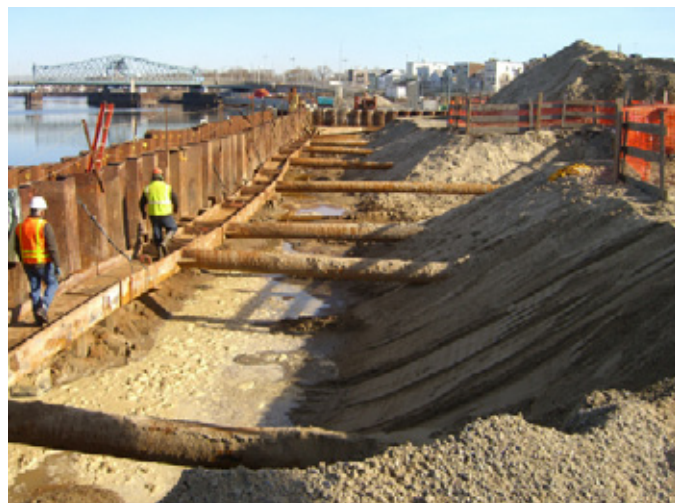
BULKHEAD RECONSTRUCTION BY ARMY CORPS
