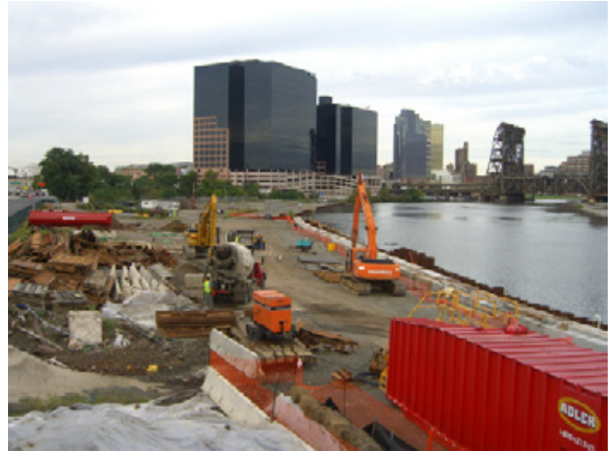
BULKHEAD CONSTRUCTION
